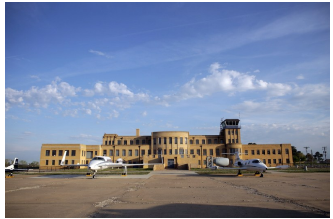
Figure 1: The main terminal viewed from the rear.
